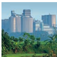
Largest cement plant of the Group: Citeureup, Indonesia
