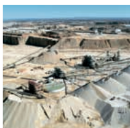
Bridgeport aggregates plant in Texas, USA
