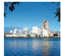
Mason City cement plant in Iowa, USA
